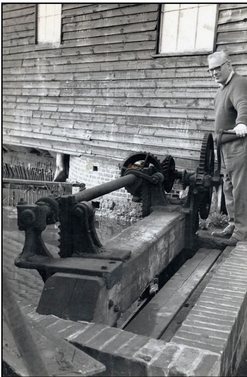
Malcolm Pummell opening the sluice gates
